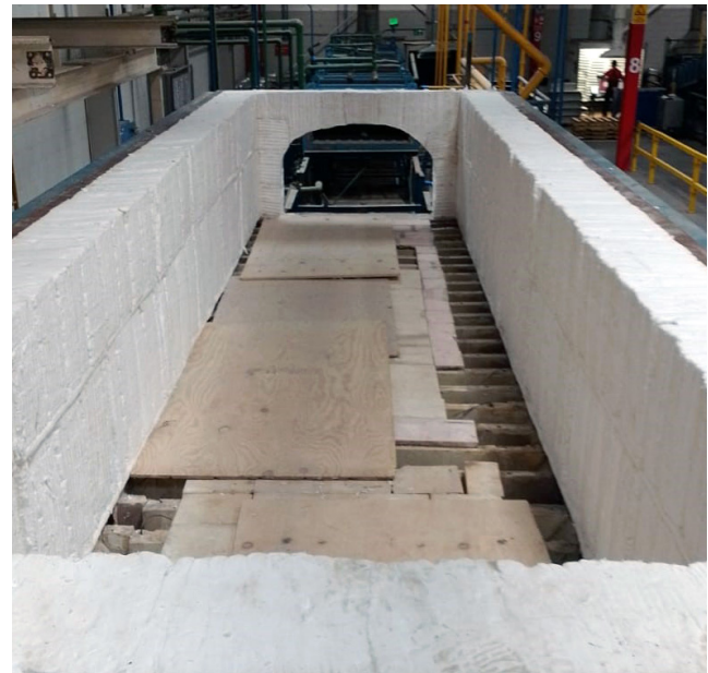
Fig.1 MaxBlock 2600 modules and MaxRigidizer stiffener application
